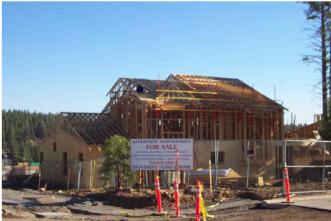
New construction activity is a significant force in the local economy
